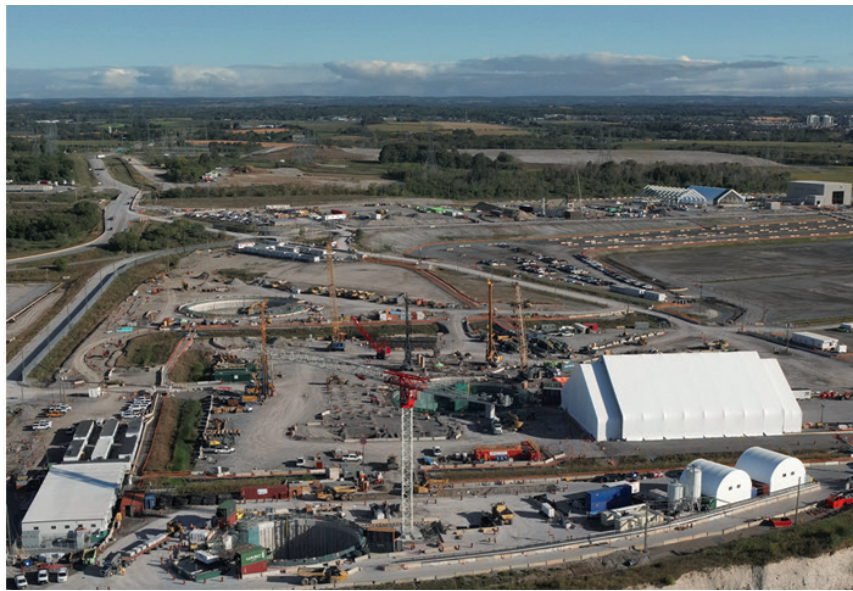
Figure 7 - Construction of GE Hitachi's BWRX-300 SMR. 11
