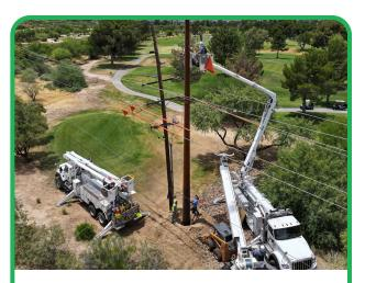
Wood and steel pole testing ensures the integrity of our equipment. In 2024, we proactively replaced 228 wood poles with steel poles, in additions to emergency restoration and system integrity replacements.
