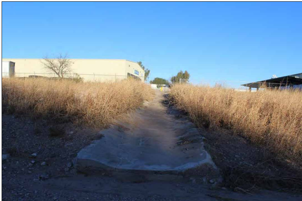
Drainage apron leading to Mariposa Canyon Wash in section 5
