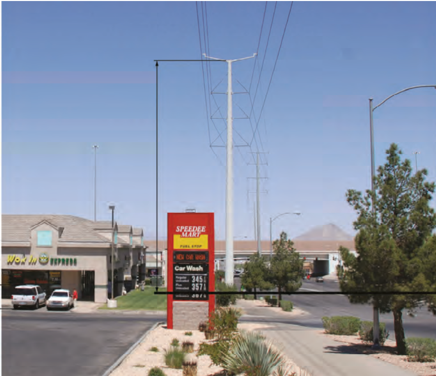
Example of the proposed 230 kV Transmission Tower (about 105' in height)
