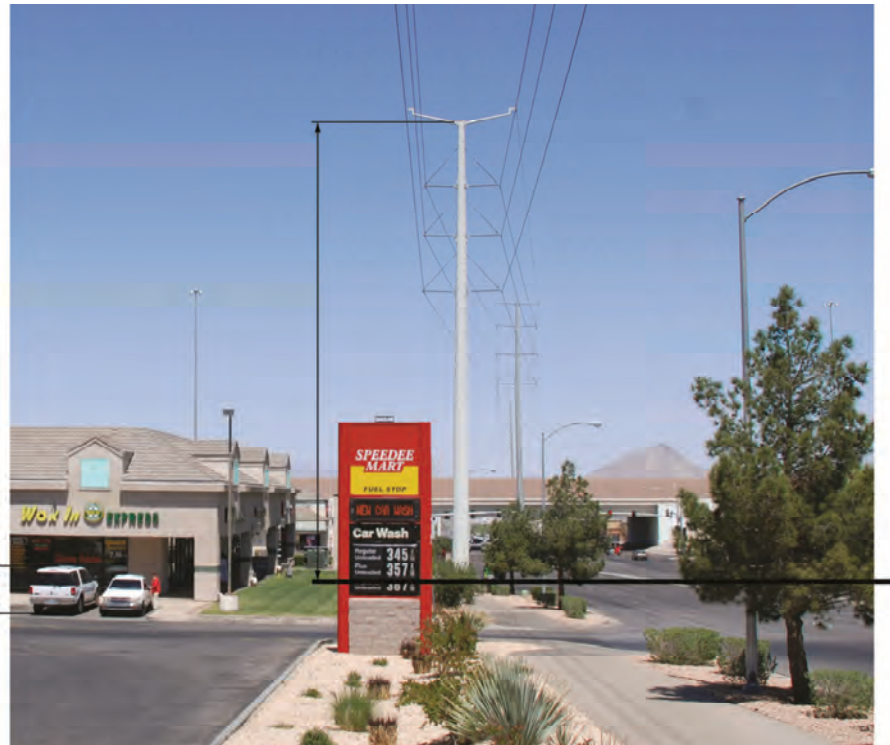
Existing 69 kV (about 50' in height) and Proposed 230 kV Transmission Tower (about 105' in height)
