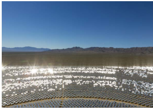
Ivanpah Computer Controlled Heliostats
