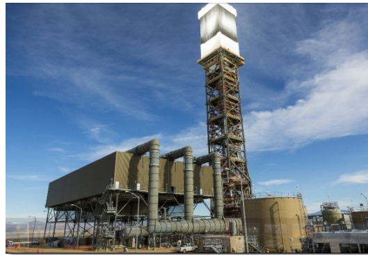
Ivanpah Solar Receiver and Condensers
