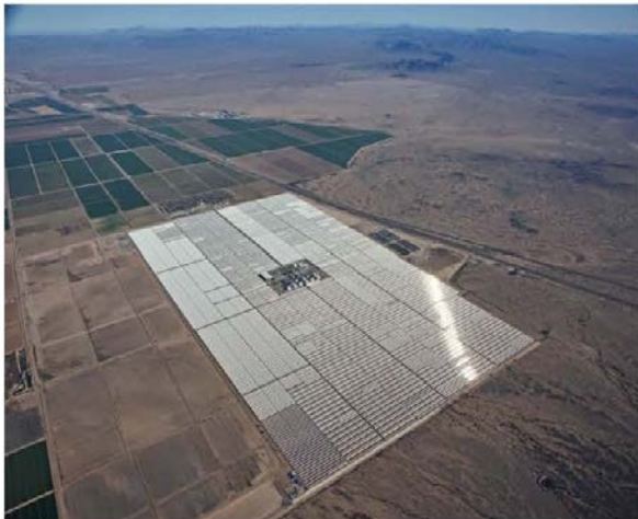
Aerial View of Solana Solar Field
