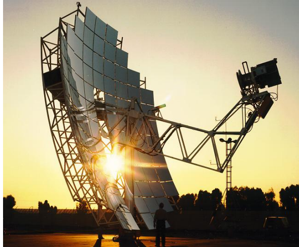
25 MW Solar Parabolic Dish-Engine System (NREL)
