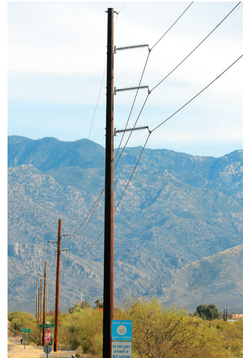
A typical weathering steel monopole supporting a 138 kilovolt transmission line.
