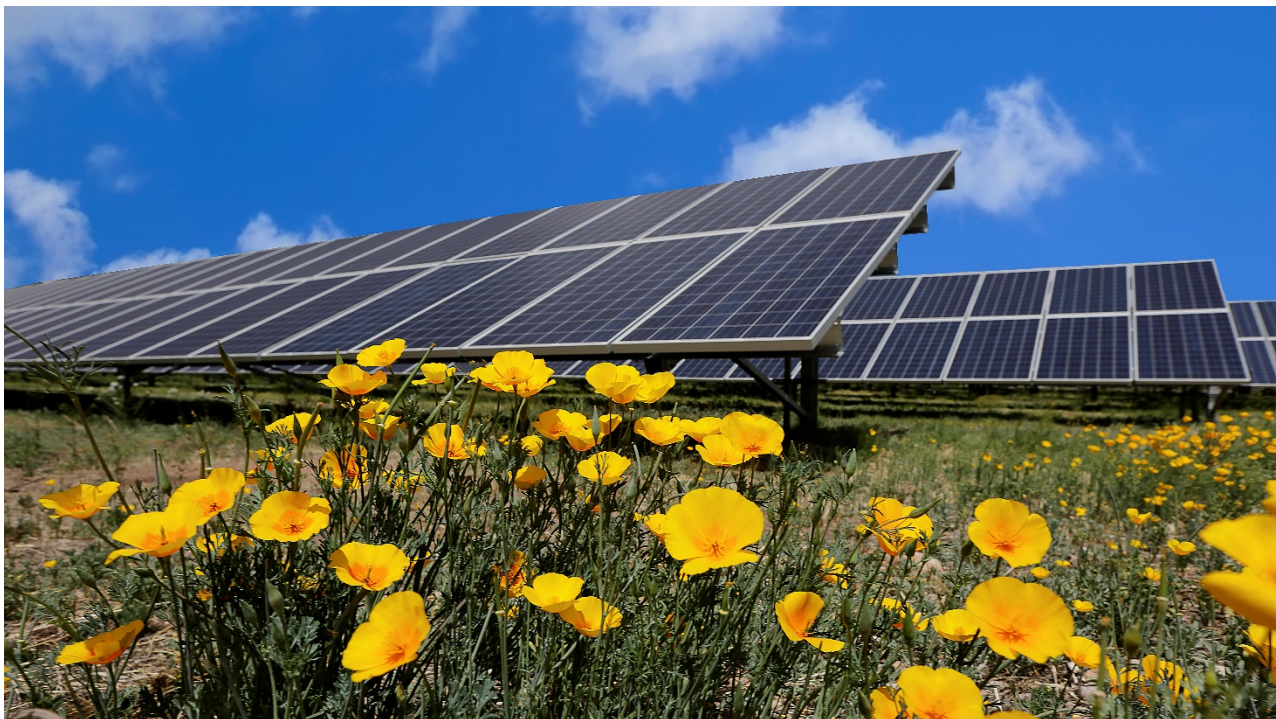
Picture 2 - UNSE Solar Facilities Located at the Rio Rico High School
